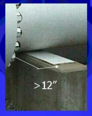
Keep weld joints at least 3" from supporting steel or other obstruction
