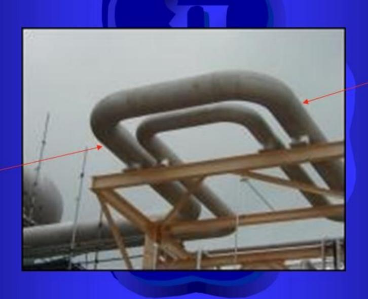
Take gas and vapor branch lines from tops of header where it is necessary to reduce the chance of drawing off condensate or sediment which may damage rotating equipment
